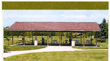
Erie Shelter at Ottawa Metro Park
